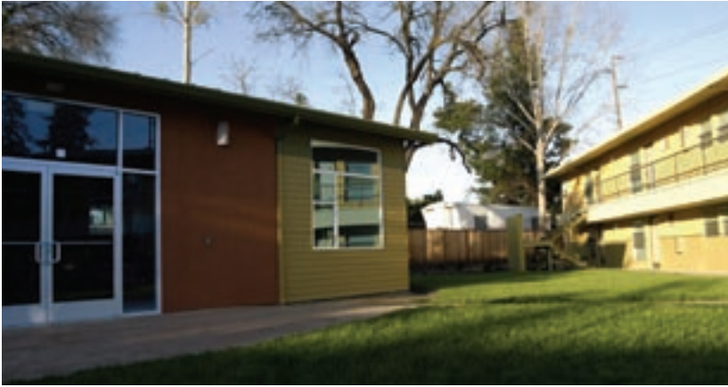
Contra Costa Interfaith Housing's Garden Park Apartments in Pleasant Hill
